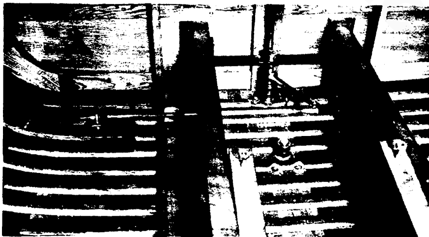
Fig. 15 Typical Bed, Stringer and Steering Set-up
